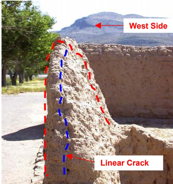
Clumping (Figure A3.8) results when wall portions that are not restrained by surrounding adobe wall mass are subjected to more water absorption. Without the restraining effect of the wall mass, the wall tops and ends can crack more severely and consequently become separated from the surrounding material, resulting in “clumps” of adobe material. The clumps are then subject to displacement by
