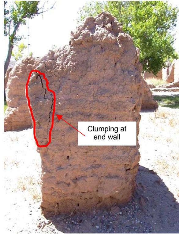
identified several areas where material recently had scaled or flaked off the wall surface. In some cases a pattern of surface cracks also are associated with the detachment, particularly on the north and east walls. The detachment indicated by sounding also exists in walls with relatively few surface cracks. The south- and
