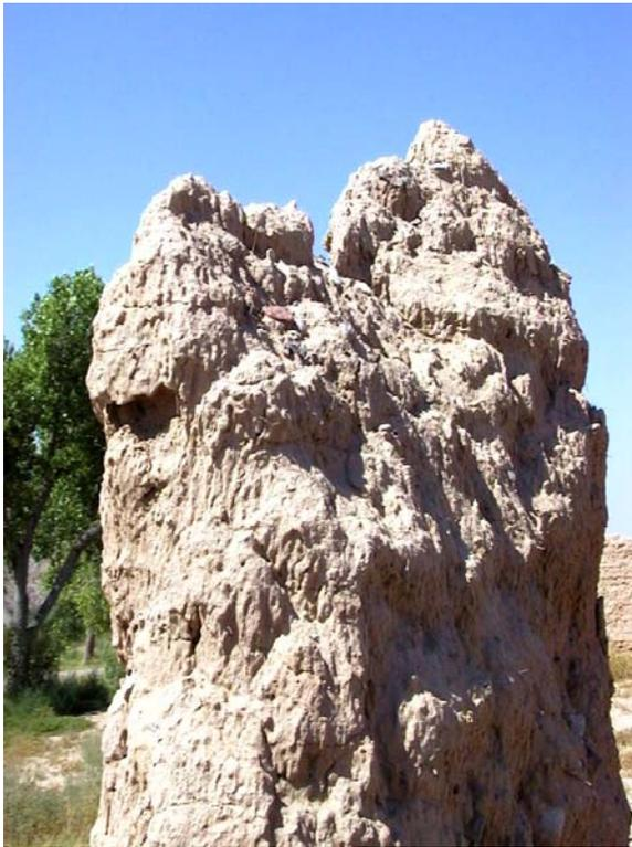
Another critical condition presently causing material loss is the detachment of adobes in layers between ½ and 2 inches thick. The condition appears to exist on all vertical wall surfaces regardless of the visual difference of the surfaces and does not appear related to the particular direction the wall surface faces. This
